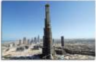
Tearing the Tower Down... Brck by Brick
