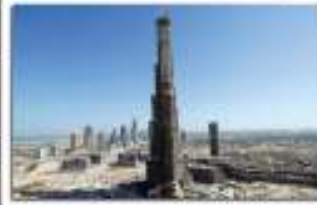
Tearing the Tower Down... Brck by Brick
